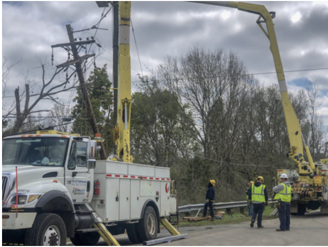
Crews begin to fix snapped power lines that have been littered by tree branches. Ila Wilborn | The Famuan
