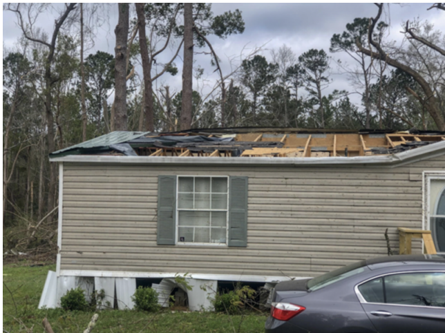
With winds reaching an estimated 140 mph in the storm's path, this homeowner's roof ripped off of her home.
